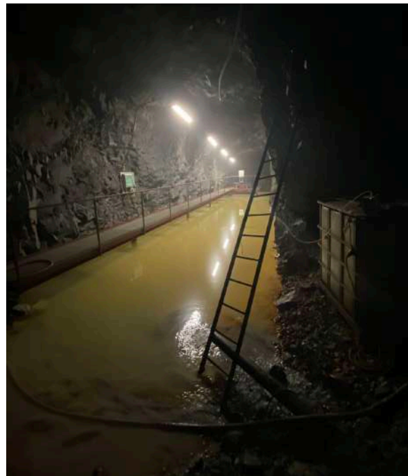
FIGURE 9. Basin for infiltrating groundwater in Lovisagruvan.
